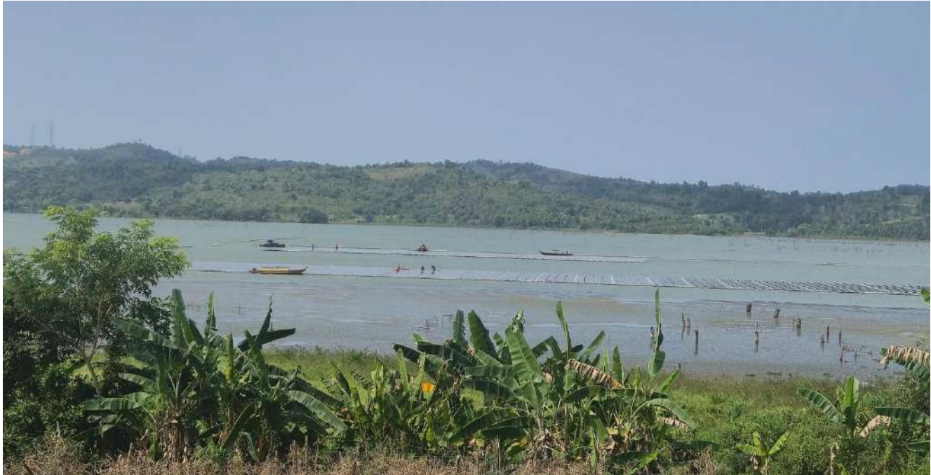
Figure 7. Documentation of the Tembesi Solar PV Construction Process
