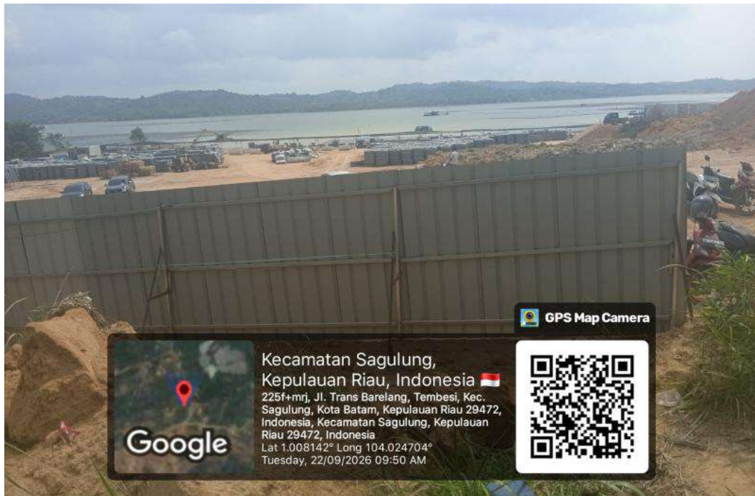
Figure 9. Documentation of Construction Progress at the Tembesi Reservoir Solar PV Project
